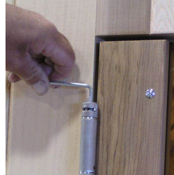
Once set pin is in place, remove wrench
