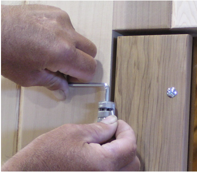
Tighten tension and insert set pin
